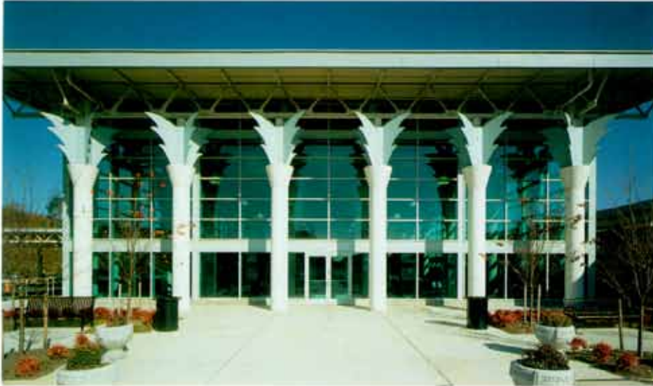
Amtrak Auto Train Location: Lorton, Virginia Products: Azuria/Solarban 60 Glass Architect: Jacobs Facilities Glazing Contractor: Engineered Construction Products Glass Fabricator: J.E. Berkowitz, LLP Owner/Developer: Amtrak Auto Train
